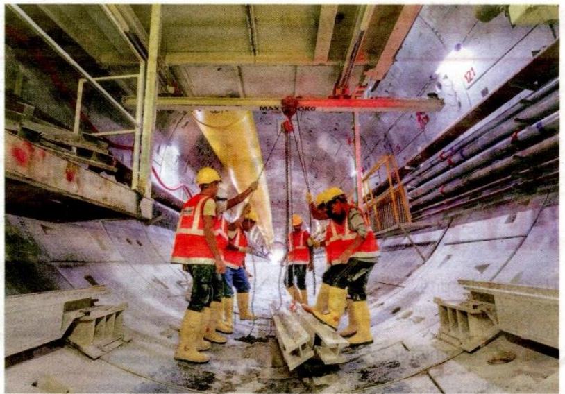
Tunnellers lifting the gantry rail beam to be sent to the front of the VD TBM at one of the MRT Line 2 worksites.
